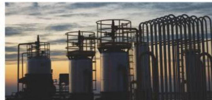
液化天然气行业 Liquefied natural gas industry
